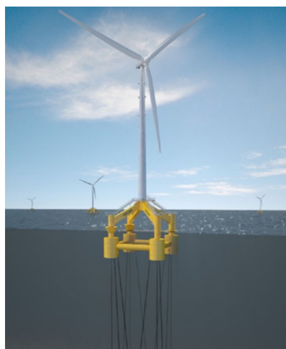
Figure 6: GICON SOF TLP substructure (GICON SOF, n.d.)
