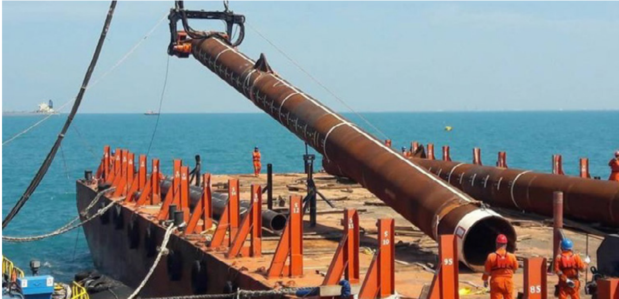
Figure 14: Driven pile anchor during deployment (Offshore Engineer, 2019)
