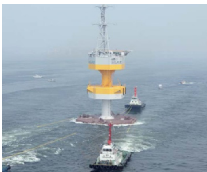
Figure 26: Fukushima floating offshore substation (Fukushima Offshore Wind Consortium, n.d.)
