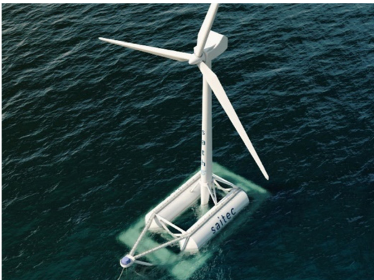
Figure 11: Saitec's DemoSATH platform, featuring a single point mooring system (Saitec, 2020)
