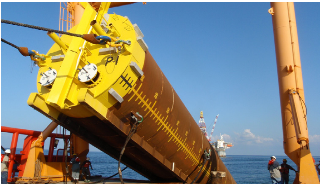
Figure 15: Suction pile anchor during deployment (Intermoor, 2021)
