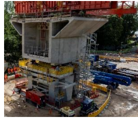
Joining pre-cast sections
