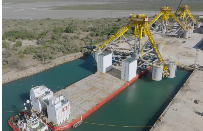
Figure 11 Provence Grand Large TLPs being stored quayside and floated off via barge [15]
