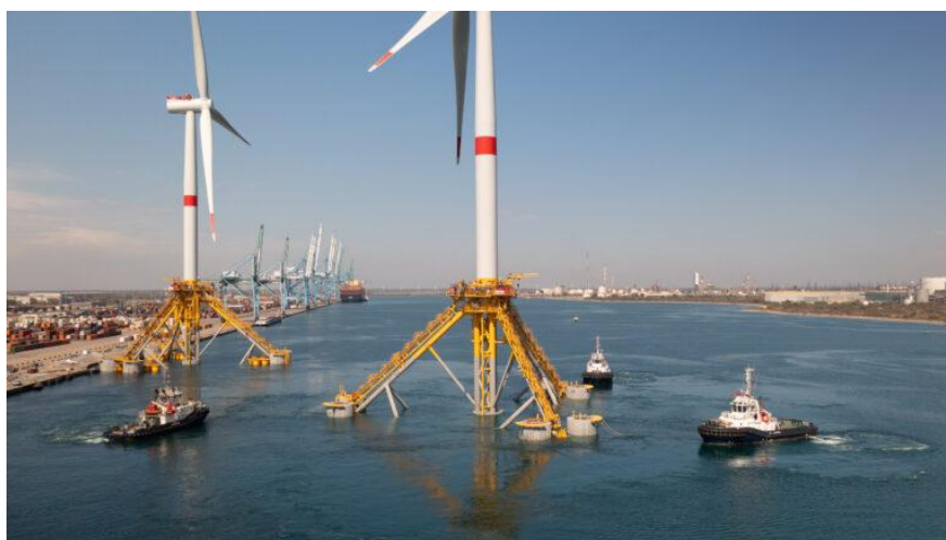
Figure 12 Provence Grand Large turbines being towed after turbine integration [16]
