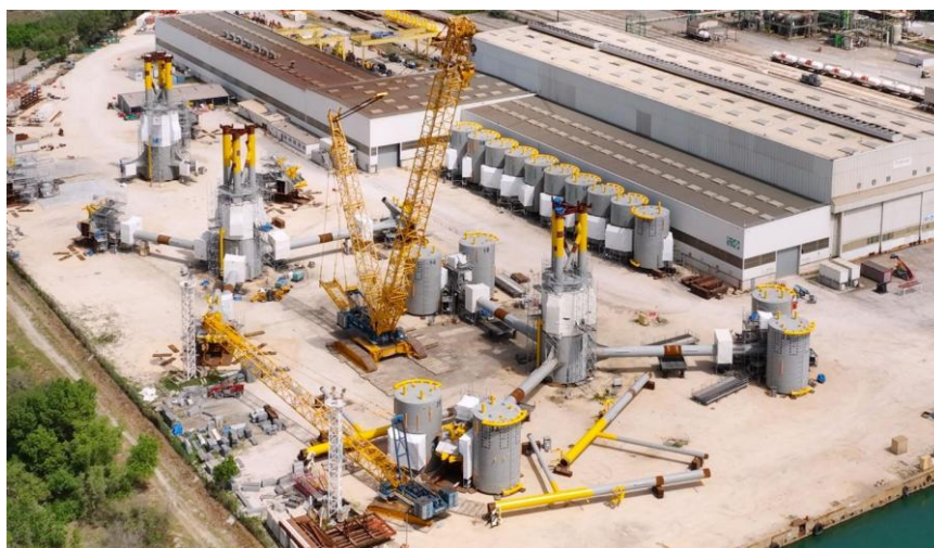
Figure 7 SBM Offshore® TLP Assembly in Eiffage Metal®'s yard in Fos-sur-Mer [13]
