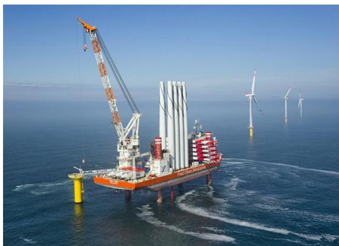
Figure 15 Jack-up vessel conducting an in-situ turbine integration for a bottom-fixed structure [17]
