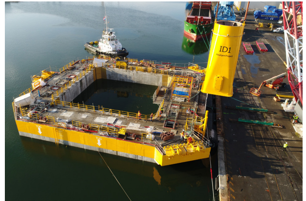
Figure 10 - Construction, Operations and Maintenance (credits: Floatgen TP - ECN S.ARCHVEQUE)
