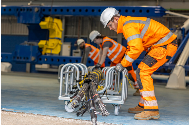
Figure 24 - Cables at the Floating Wind Innovation Centre in Aberdeen (credit: ORE Catapult)
